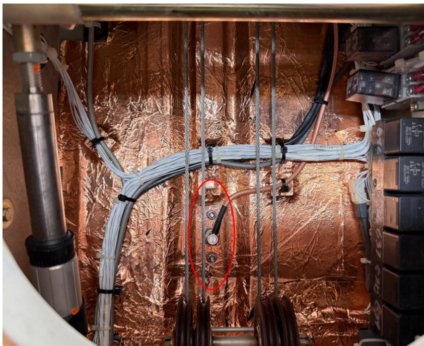
Figure 6: G1 Antenna Installed with Ground Plane
